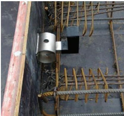
HLDQ-L30 Sleeve nailed to formwork
