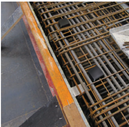
Reinforcement around ESDQ-L20 Sleeves
