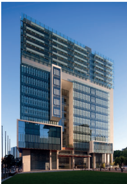
2,500 Lockable dowels were installed on the Supreme & District Court, Brisbane, QLD
