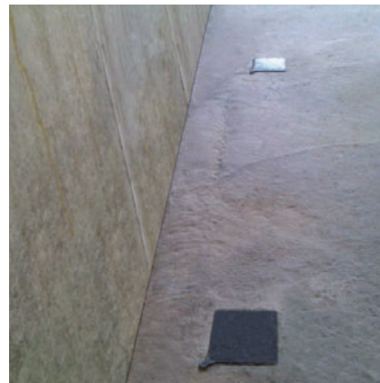
Void formers shown at Slab-to-Wall joint
